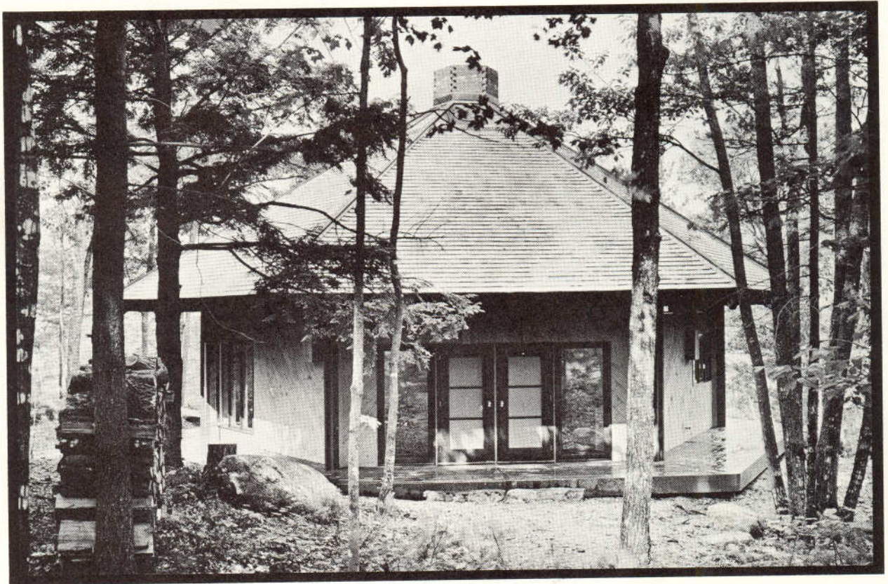
View of the front entrance to the "Sundown," one of the vacation homes designed by architect-developer Delnoce Whitney Goubert for "Oakledge" in the Dartmouth-Sunapee region of New Hampshire. Exterior siding is of natural wood for minimum maintenance.
